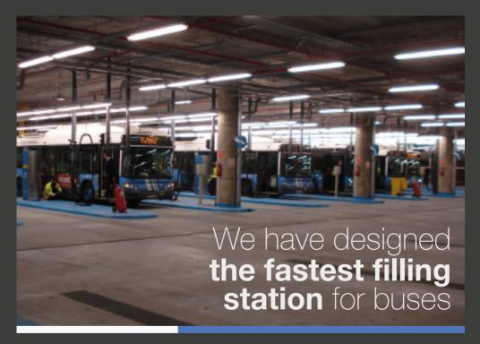
We have designed the CNG filling station of the Sanchinarro Operations Center, which belongs to Madrid's Municipal Transport Company (EMT) in Spain. Cutting-edge technology makes it possible to refuel between 150 and 180 buses per hour by means of Coldbox® and Common Manifold® direct filling, entirely developed and manufactured by Galileo.
