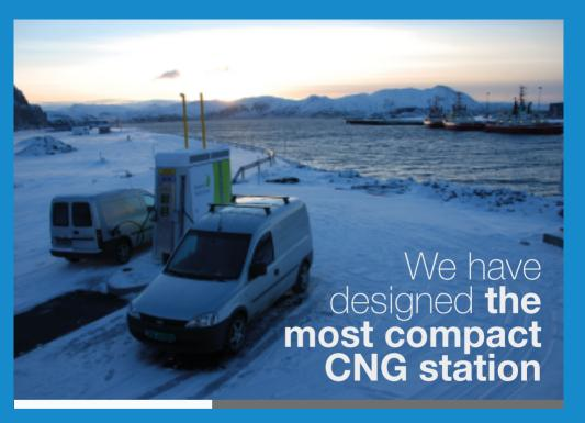
Our Nanobox® packaged CNG station has offered an innovative solution to drivers in the Norwegian city of Hammerfest, the northernmost city in Europe. In one single compact module we integrated compression, storage and dispenser.
