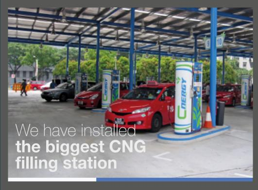
In Singapore, we combined our Microbox® CNG packaged compressors and our EMB® dispensers to refuel 46 cars simultaneously. We have also achieved a remarkable record: according to Guinness World Records, this is the largest CNG station worldwide.
